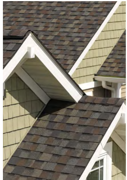
ROOFING AND VENTILATION
