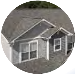
Roofing and Ventilation
